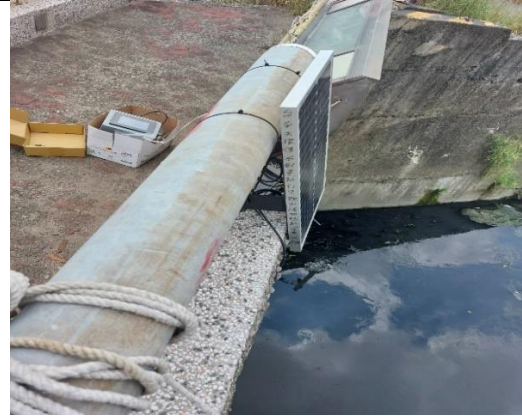
Solar panel installation status
